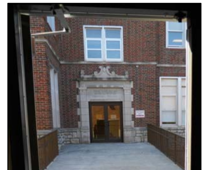
This is a walkway from mid-east entrance into Junior High main building. A walkway and banister has been constructed for safer travel and access into FEMA building.
