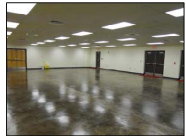
Another FEMA area to the west of the gym and north of the cafeteria
